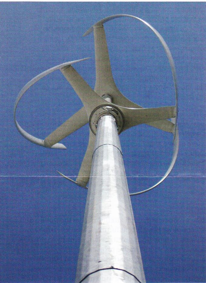
turbines—vertical axis turbines that capture wind from all directions and can generate power at a higher level of productivity. The turbines are especially suitable for use in urban areas and can supply enough energy to power a home or small office building.
