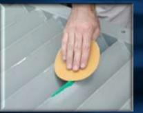
When base coat is fully dry/cured (approx.4hrs), sand area with 100 grit to feather in and remove all shine
