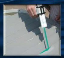
Pull trigger of gun applicator and apply base coat to affected area. If desired paint may be spread with a foam brush
