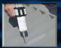
Pull trigger and apply top coat to affected area. If desired paint may be spread with a foam brush.
