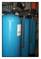
The ultra clean water is actually corrosive to mild steel. Everything must be built from plastic, stainless steel or epoxy coated steel.
