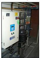
This state of the art R.O system can produce up to 15 GPM 24 hours a day.
