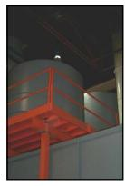
2 2500 gallon plastic R.O water tanks give ACL lots of capacity & flexibility.
