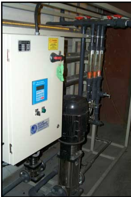
This state of the art R.O system can produce up to 15 GPM 24 hours a day.
