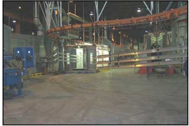
Extrusions are entering the spray booth for the electrostatic powder coating.
