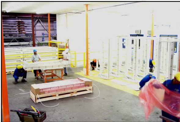
Final Inspection, wrapping in anti-static bags & packaging on the skids for direct shipment to end user.
