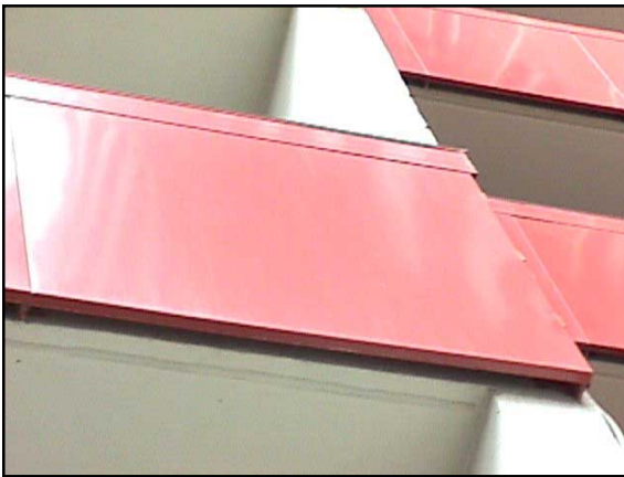
Over two years in service the finish remains clean, maintenance free with a gloss retention of 96%
